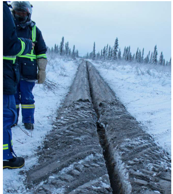
Quality assurance review of trench depth.
