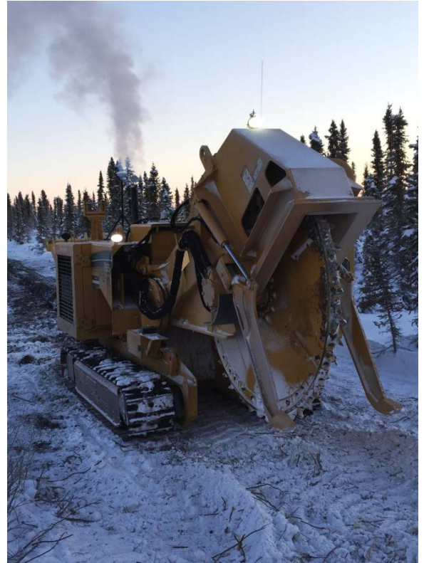
A T555 saw cutting the cable trench south of Inuvik.
