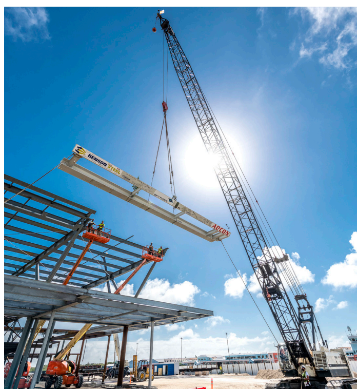
The last piece of structural steel for the new terminal building is lifted into place in September 2018.
