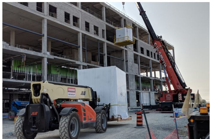
A crane lifts one of the modular washroom pods while another waits to be unloaded. The pods were 95 per cent complete upon delivery to the hospital site.
