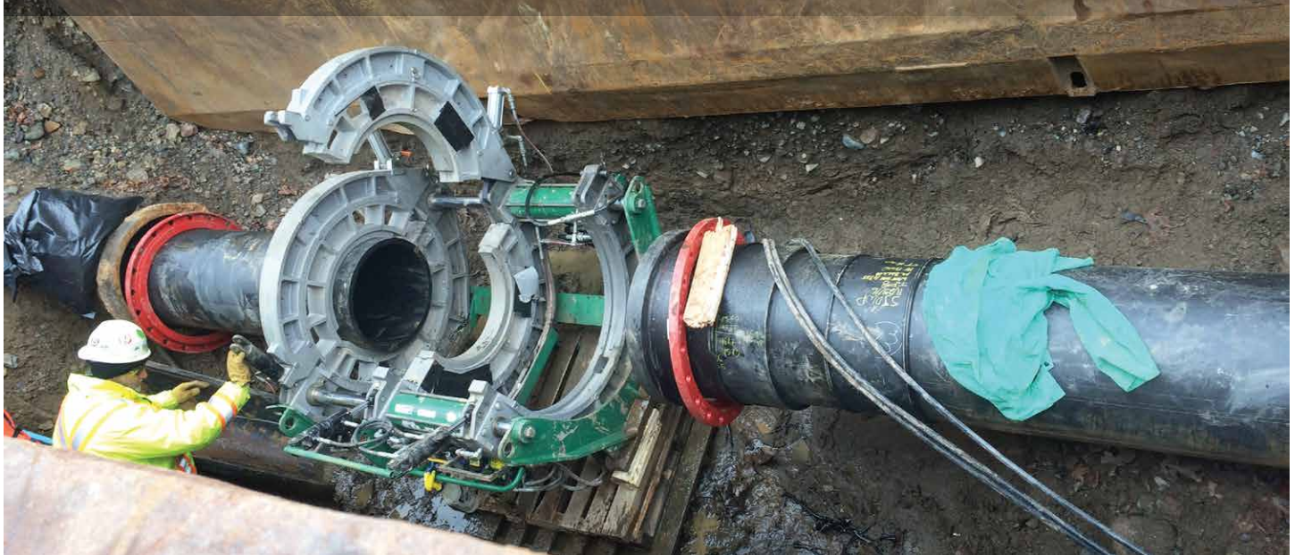
Ocean Westway sliplining of existing transmission main
