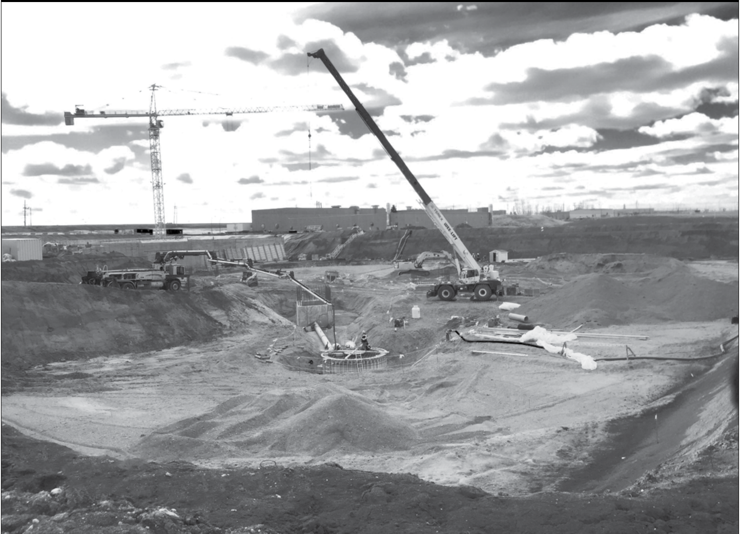
Construction of the clarifier in April 2015
