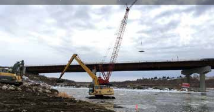
Photo 11: Hoisting prefabricated deck panels
