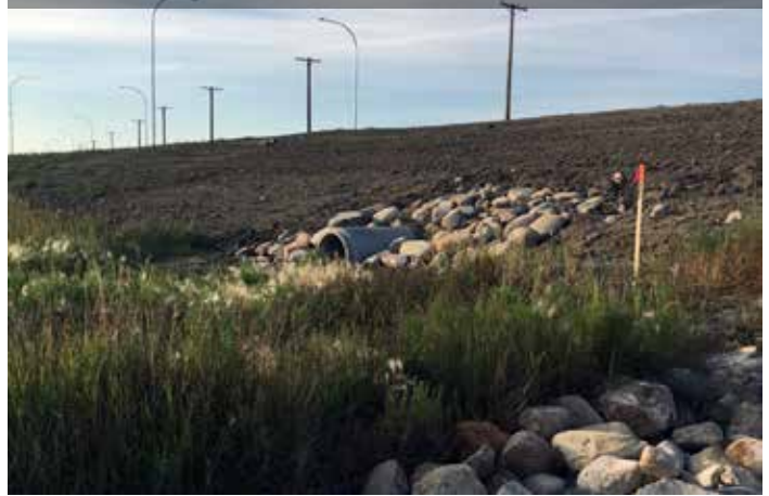
Photo 10: One of six swale-crossing culverts
