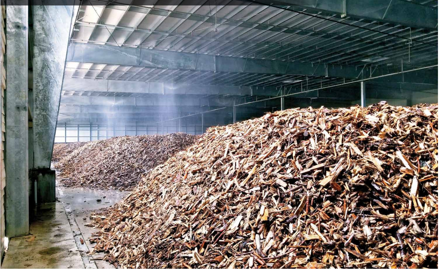
Figure 4: A critical component of the Calgary Composting Facility's odour management is its wood-chip-based biofilter
