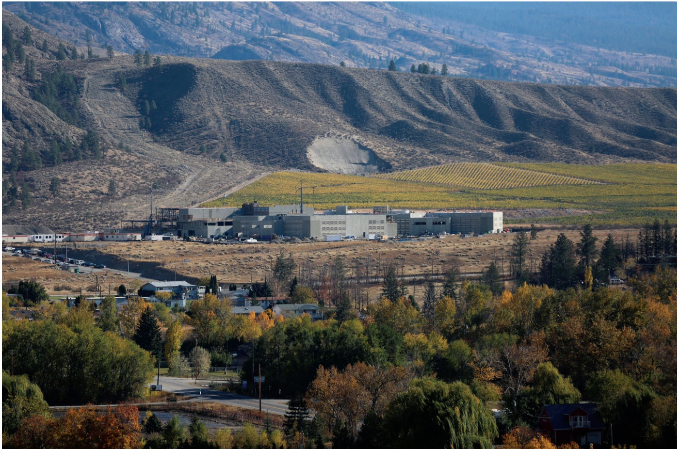
OKANAGAN CORRECTIONAL CENTRE, BRITISH COLUMBIA
