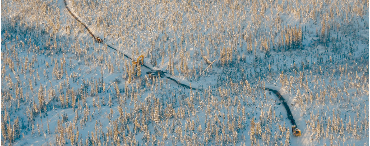
MACKENZIE VALLEY FIBRE LINK PROJECT, NORTHWEST TERRITORIES
