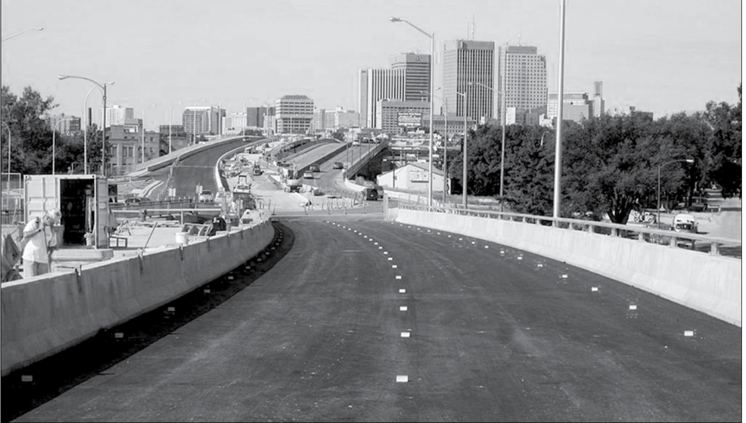
View looking west across Disraeli Bridges under construction
