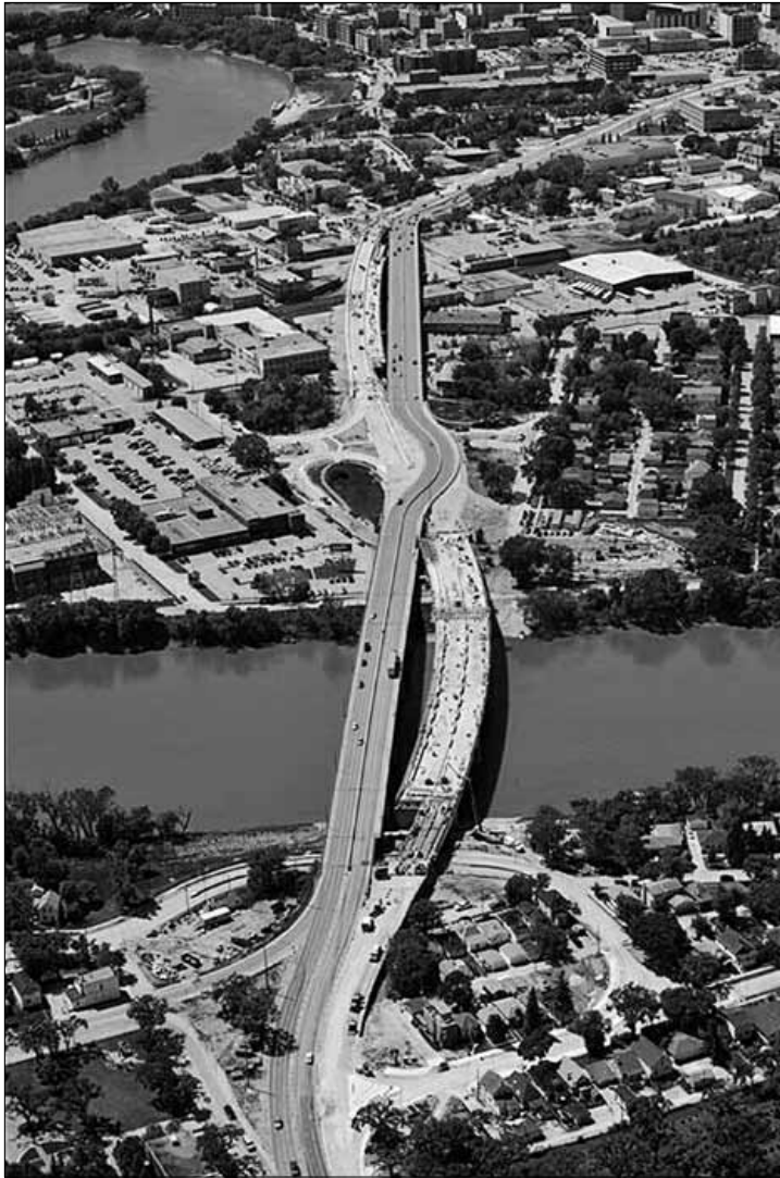
Figure 2: Aerial View During Construction
