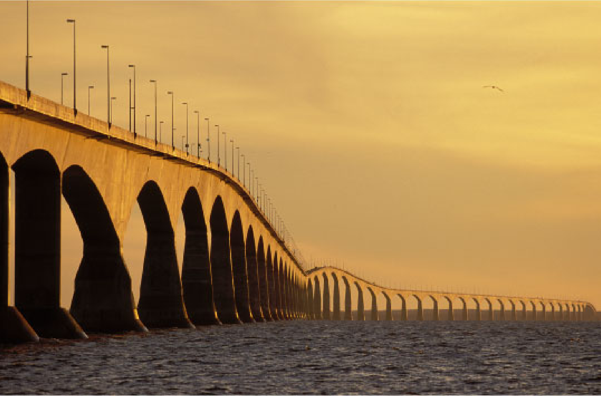
Confederation Bridge, New Brunswick - PEI
