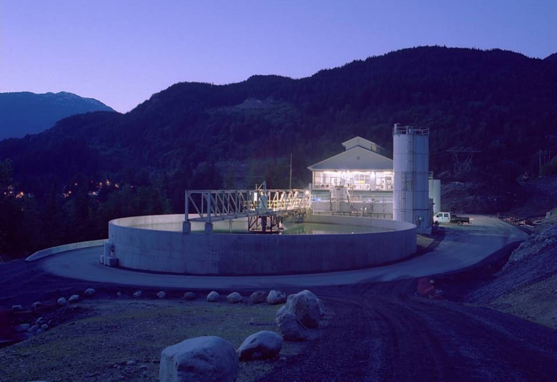
Britannia Mine Water Treatment Facility
