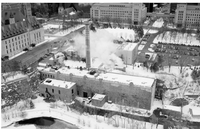
The Cliff Plant (centre) is located west of the Supreme Court of Canada in downtown Ottawa. In 2020, the Innovate Energy team demolished the 69-year-old vacant boiler room (on the right of the building). The adjacent chiller plant, constructed in 1916, will remain in operation until the first phase of the new Cliff Plant is built by late 2023.
